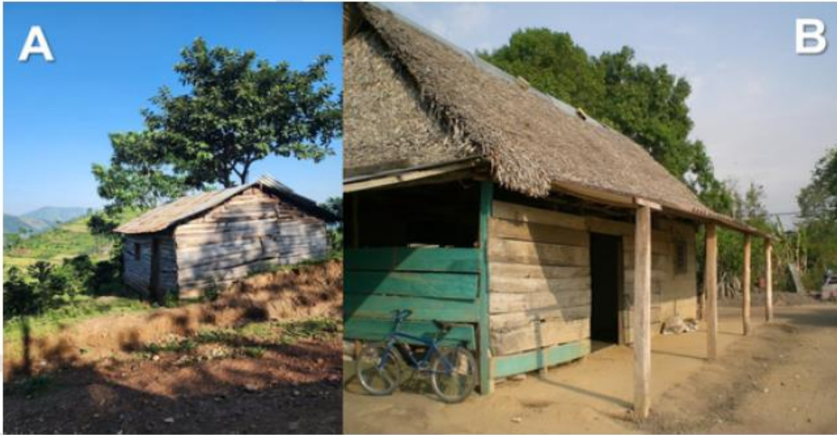
Fig. 4. Inadequate housing in rural Uganda (Bwindi) (2024) (A) and rural Venezuela (Barinas) (2007) (B). Photos taken by AJ Rodriguez-Morales.
